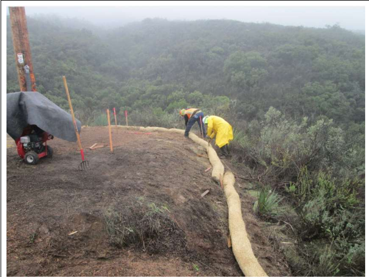
Photo 1: Crews were observed installing and maintaining SWPPP BMPs along TL 625B (fiber rolls at Pole Z272883, above).
